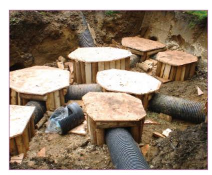
An example of an artificial sett under construction, with pipe tunnels and eight chambers.
