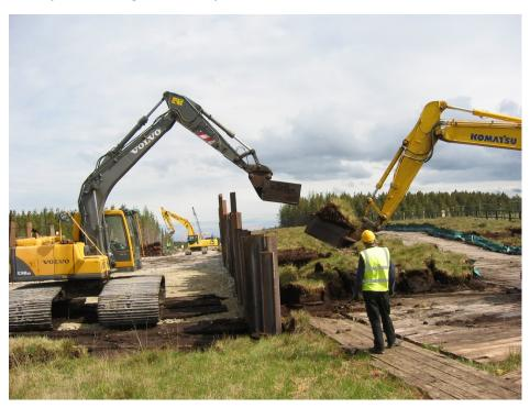
iii. Turve storage on bogmats (on RHS of sheet piled haul road and trench section on left)
