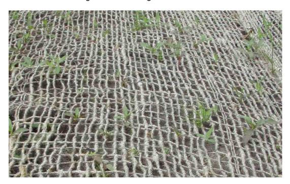
2. Use of Geojute with vegetation establishing on Landfall Valve Instiallion side slopes
