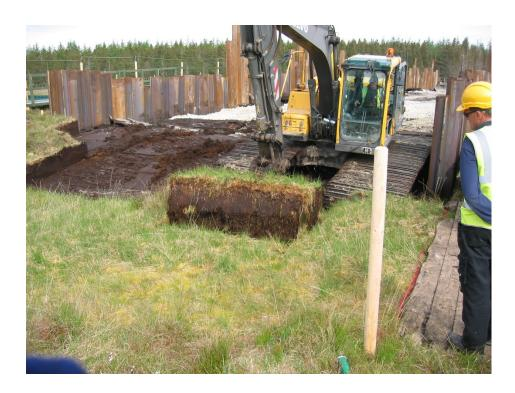
ii. Then transferred from the 'lifting' machine's bucket to the machine placing turves on bogmats in the adjacent storage area – required excellent driver coordination and care.
